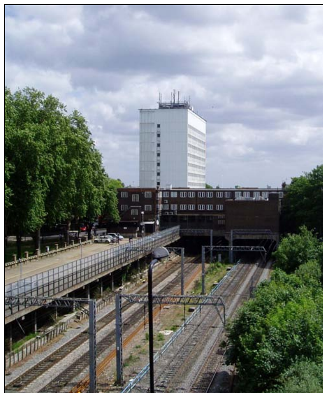
Villiers House from Springbridge Road car park, showing railway lines to be decked over in the Glenkerrin proposals. The trees of Haven Green are on the left.
